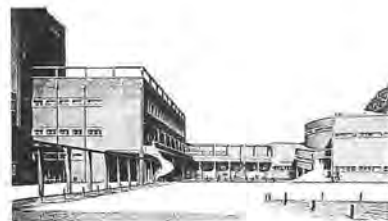
EX-GIL, Originalzustand/foto storica
